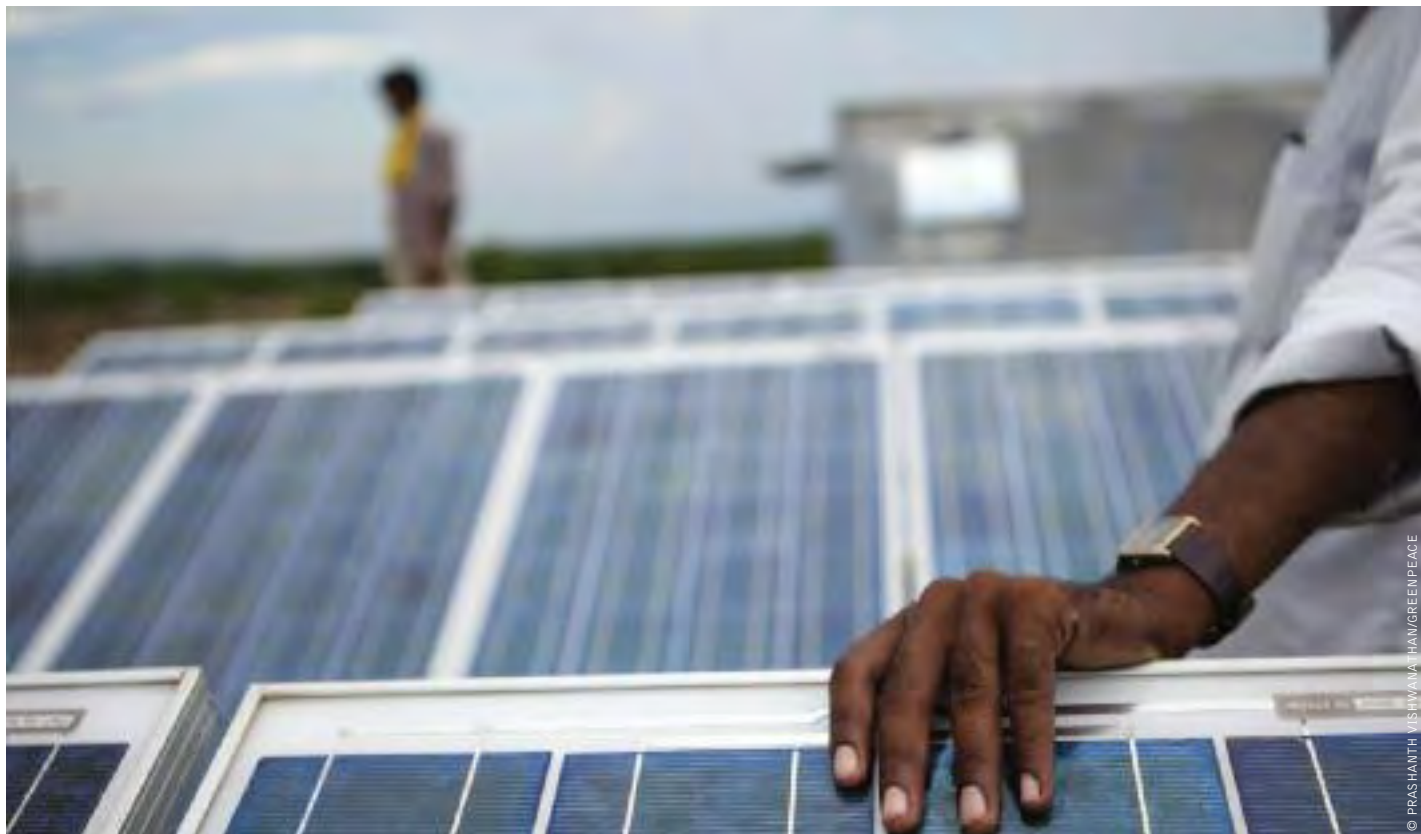
image A SOLAR-POWERED REVERSE OSMOSIS PLANT IN KOTRI VILLAGE, RAJASTHAN, WHICH PRODUCES OVER 3000 LITRES OF DRINKING WATER PER DAY FROM THE BRACKISH GROUNDWATER.
